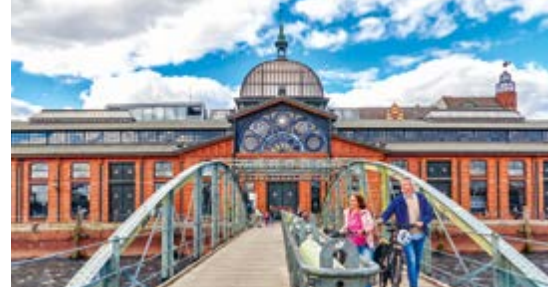
Fischauktionshalle in Altona ▶
